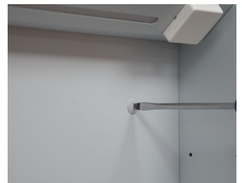
Step 4 - Lock securely in place * Different locking systems apply to mirrors and cabinets
