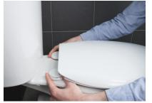
**ALIGN**Align the hinges to the toilet pan and push hinges in place.
